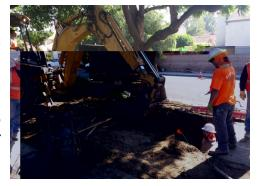
Just before and between two planned power outages in August, crews from Tidwell Excavations, SCE's contracted company, redesigned and replaced an aging power switching station alongside Sterns Ave. The new equipment will minimize future brown-outs and will ensure adequate power distribution.
